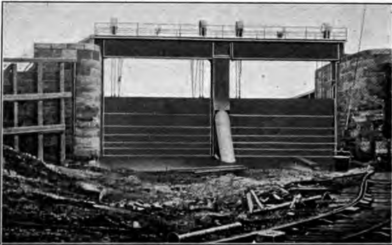
FIG. 290.—Stoney gates, Manchester ship canal.
